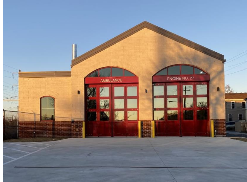
Engine Company #27 Fire Station
